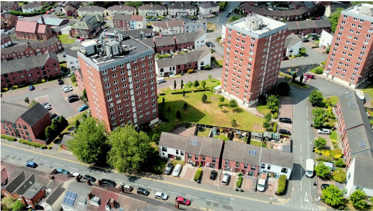
Hurcott Road high rise flats, Kidderminster
